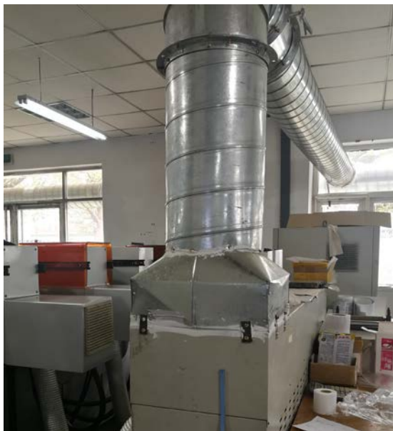
3#印刷生产线集气罩
